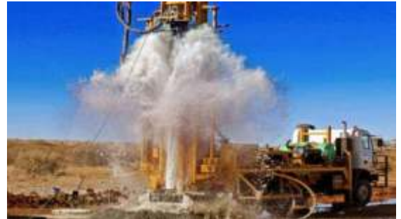
Bore Hole Construction
